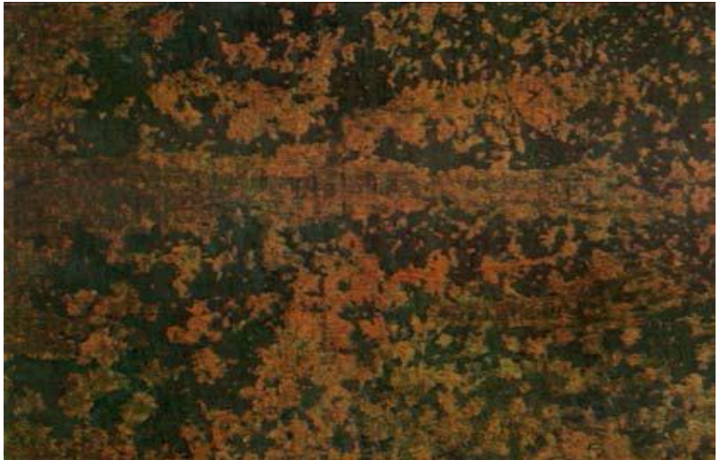
Preparation Grades. Scraping and wire-brushing B St 3
